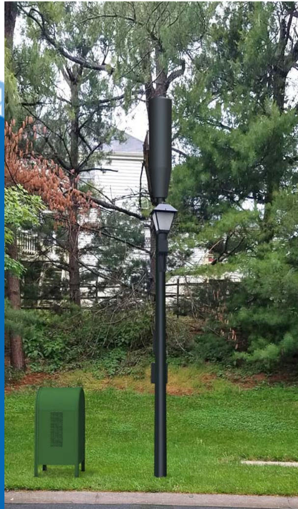
14' to 16' Colonial Streetlight Replaced with 19' to 20' side mounted or ground cabinet
